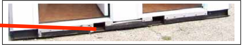
Fig. 2 - Tine Ports (Steel Frame)
